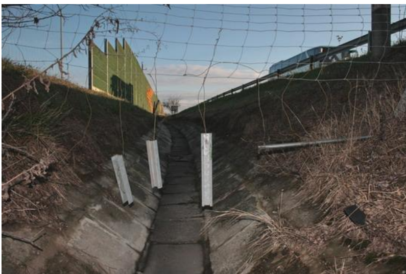
Figure 5. M1, 21 kmsz: Gap in a drainage tunnel causes high traffic safety risk because larger animals can enter to the ROW across it. The hanged pieces of metal do not prevent the entering of animals.
