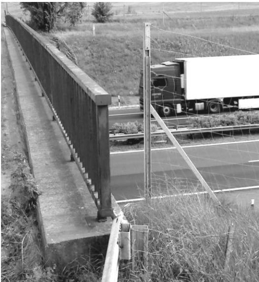
Figure 2. Fox kills are frequent at passages. Here the gaps, through which animals can enter the road, must be closed; the wildlife fence should be elongated in order to prevent animals from getting inside.
